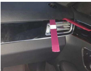
5. Pry the buckles, and remove the air conditioning panel
