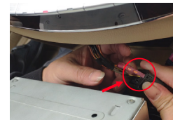
12. Take out the fiber optic cable on the original car main line
